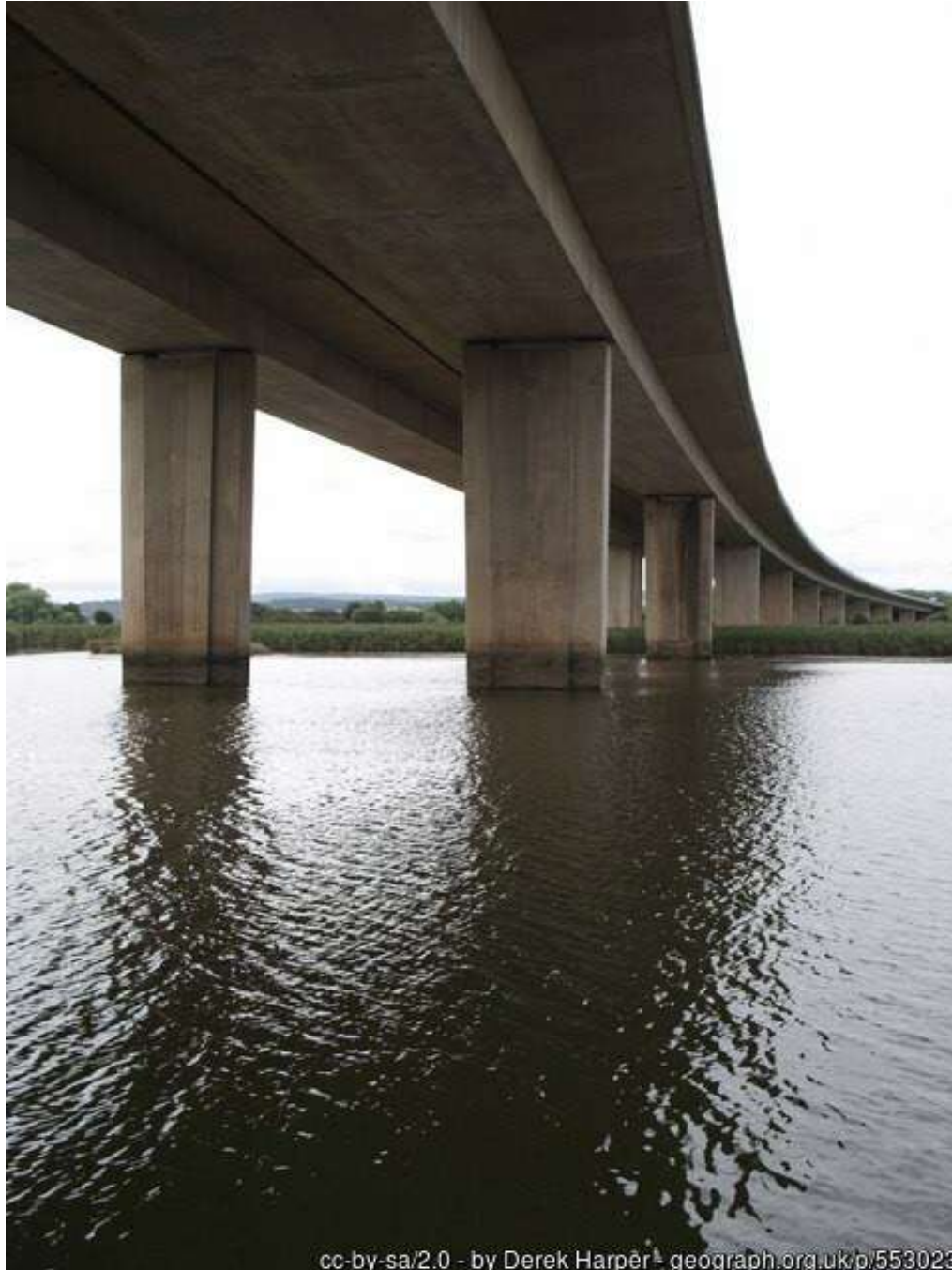
Figure 2-6: M5 Viaduct over River Exe
