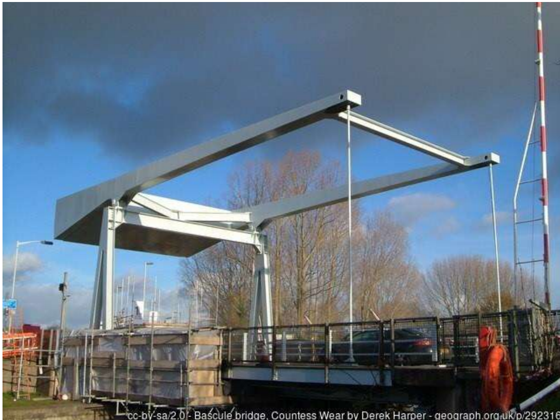
Figure 2-18: Canal bascule bridge
