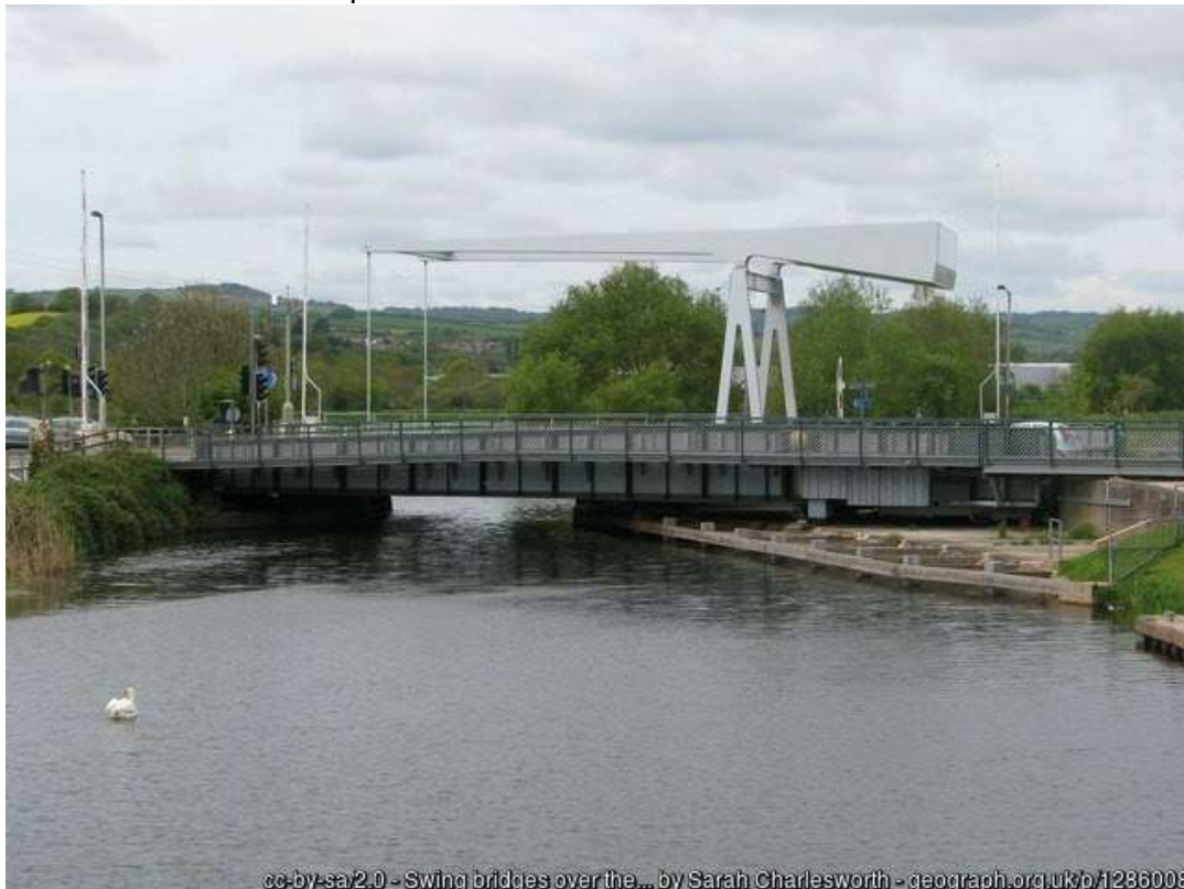
Figure 2-19: Canal swing bridge can we get a better photo
