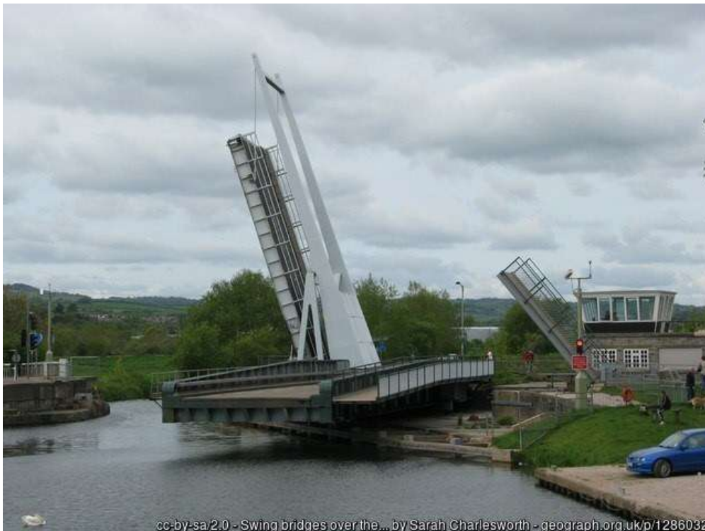
Figure 1-1: Bridge Road canal bridges, with swing bridge in foreground and bascule bridge in background.
