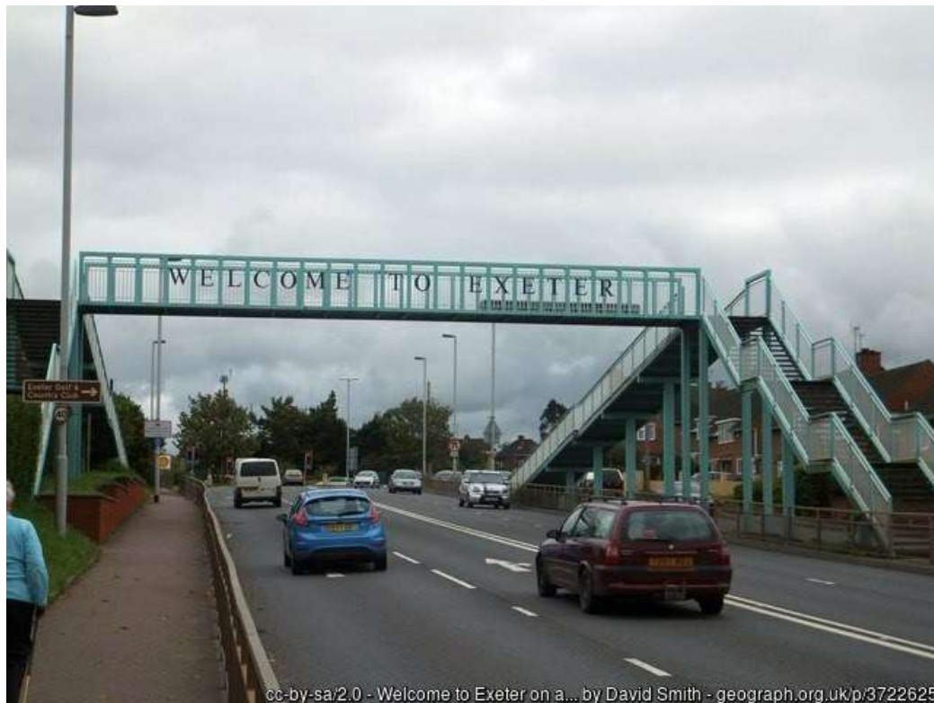
Figure 2-20: Countess Wear pedestrian bridge
