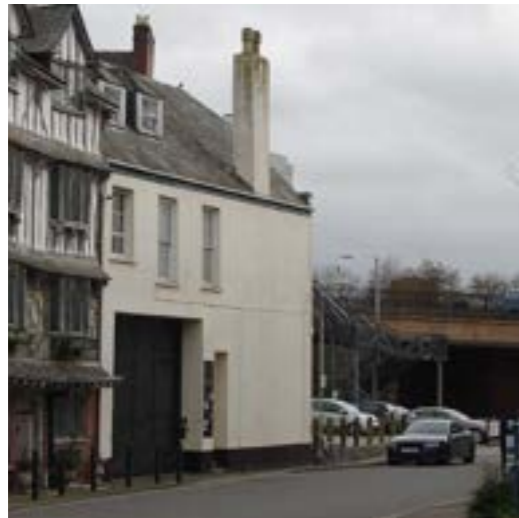
Grade II listed Eagle House. 2 and a half storey building with a rendered facade and pitch slate roof.
