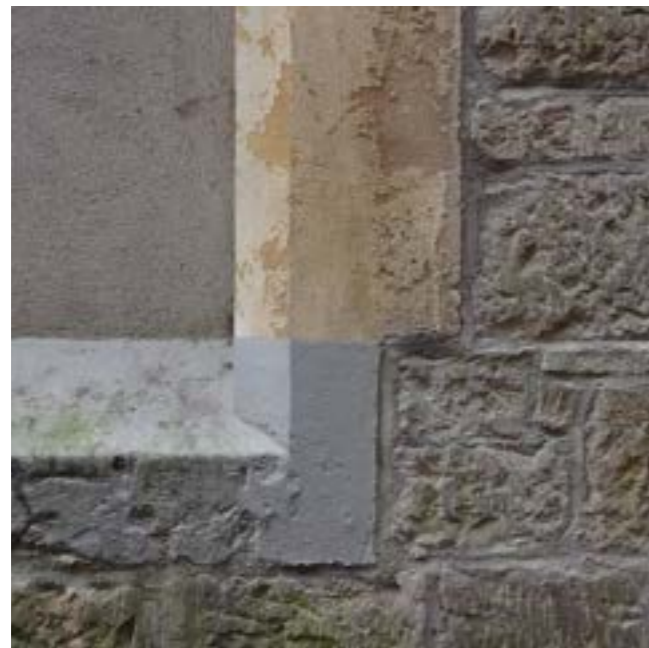
Top: Main entrance from Hick's Court. Bottom: Stonework detail showing the original stonework, blocked window and painted sill.
