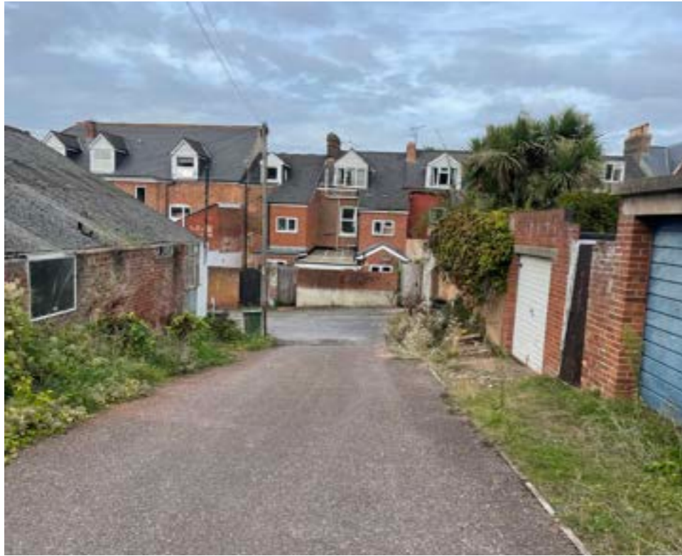
View west from within the site existing garage on the left
