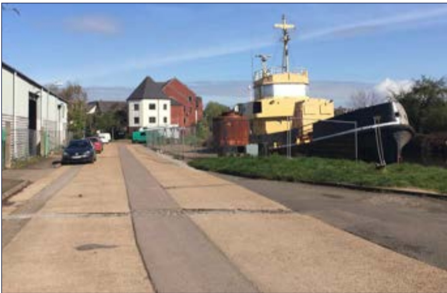
Figure 3.11: Photograph 07 - Water Lane looking River Meadows buildings
