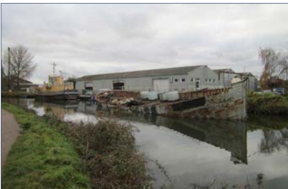
Figure 3.12: Photograph 08 - Looking towards former Coastal Workboats buildings
