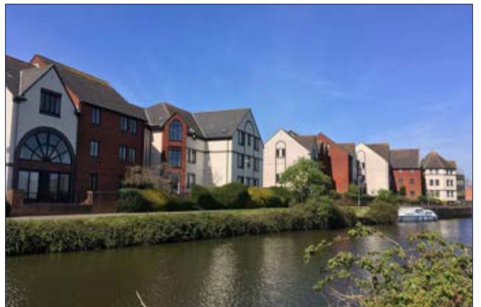
Figure 3.30: Context Photograph - River Meadows/Gabriels Wharf buildings
