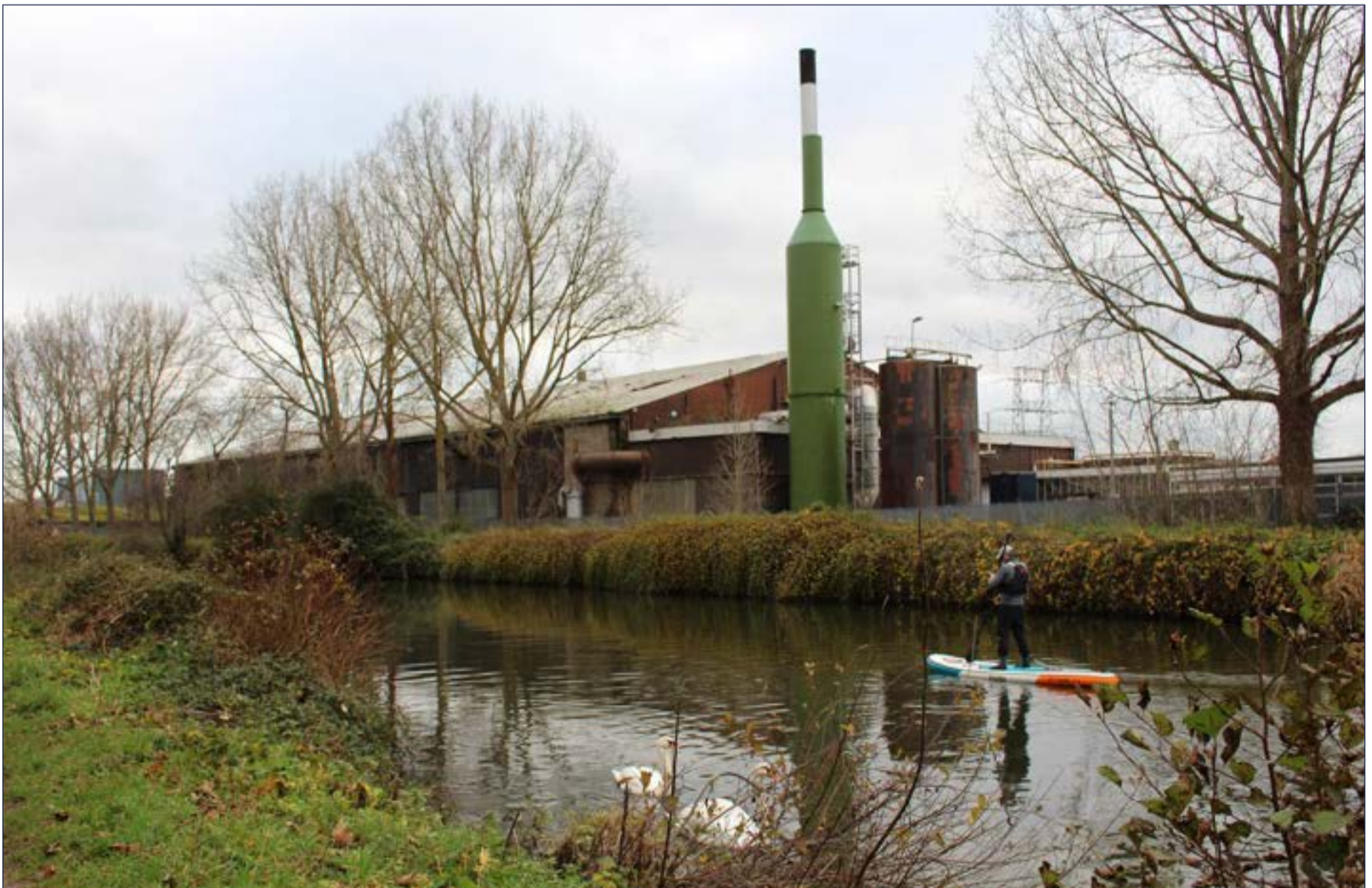
Figure 6.14: Photograph of Metal Saria Chimney
