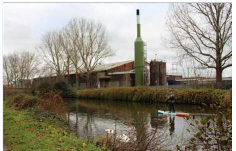
Figure 3.8: Photograph 04 - Former Saria building to south-east of site
