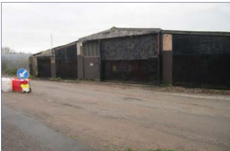
Figure 3.5: Photograph 01 - Existing building to south-east of site
