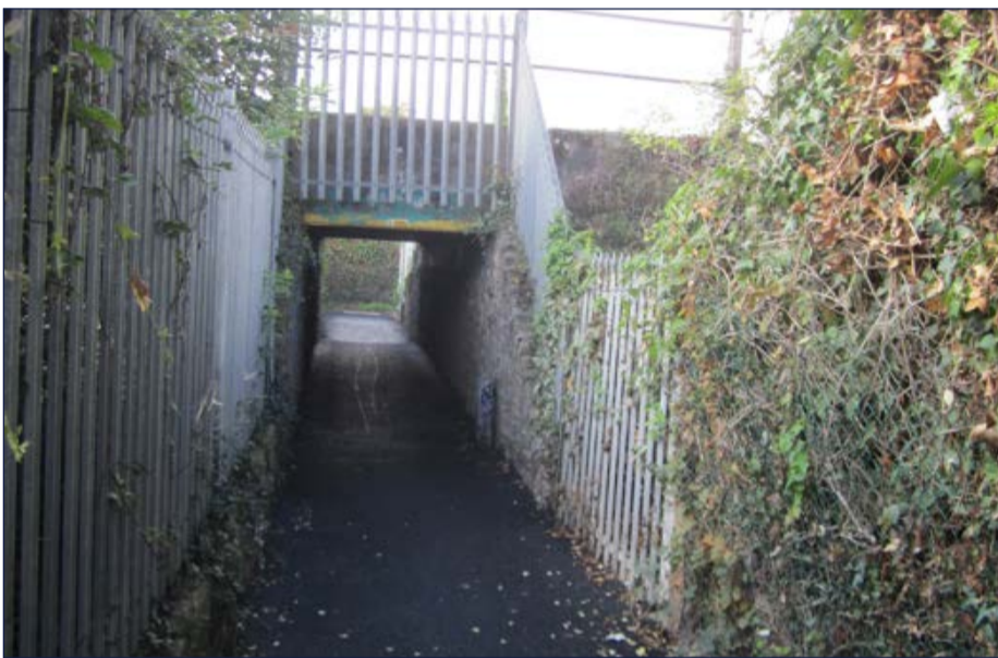
Figure 3.10: Photograph 06 - Existing railway underpass towards Marsh Barton
