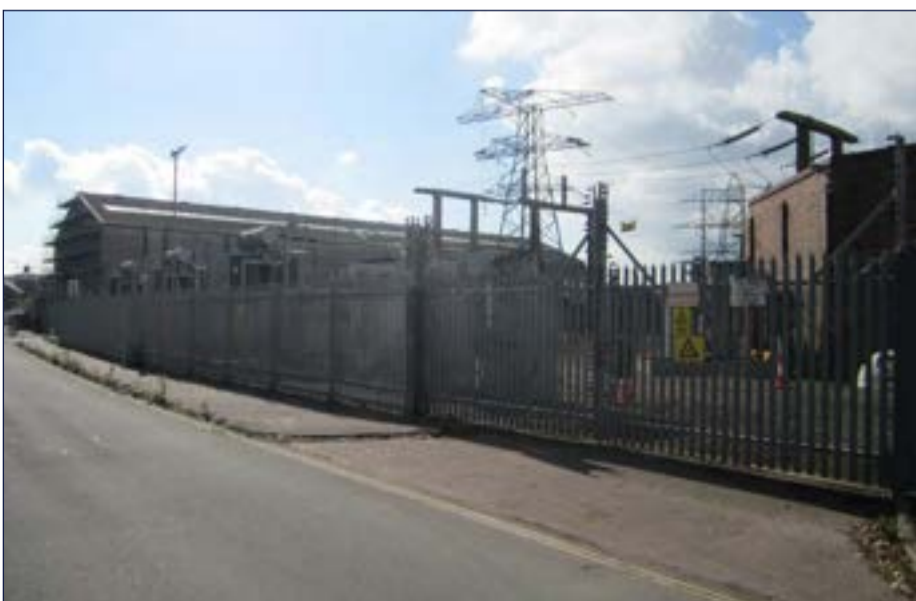
Figure 3.20: Photograph 16 - Electricity Distribution Site
