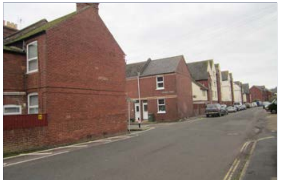
Figure 3.31: Context Photograph - Cotfield Street/Gabriels Wharf buildings
