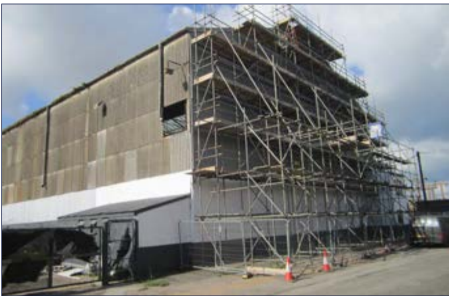
Figure 3.18: Photograph 14 - Existing building opposite Cotfield Street
