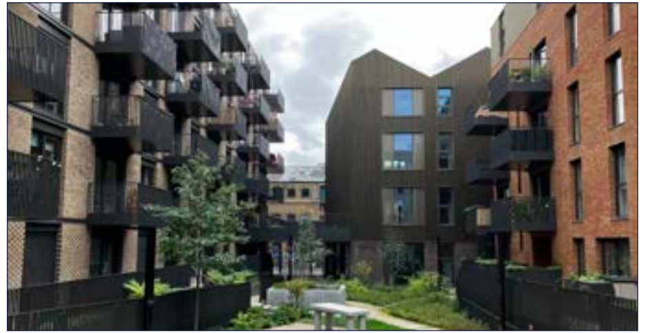
Figure 5.17: Photograph of Neptune Wharf
