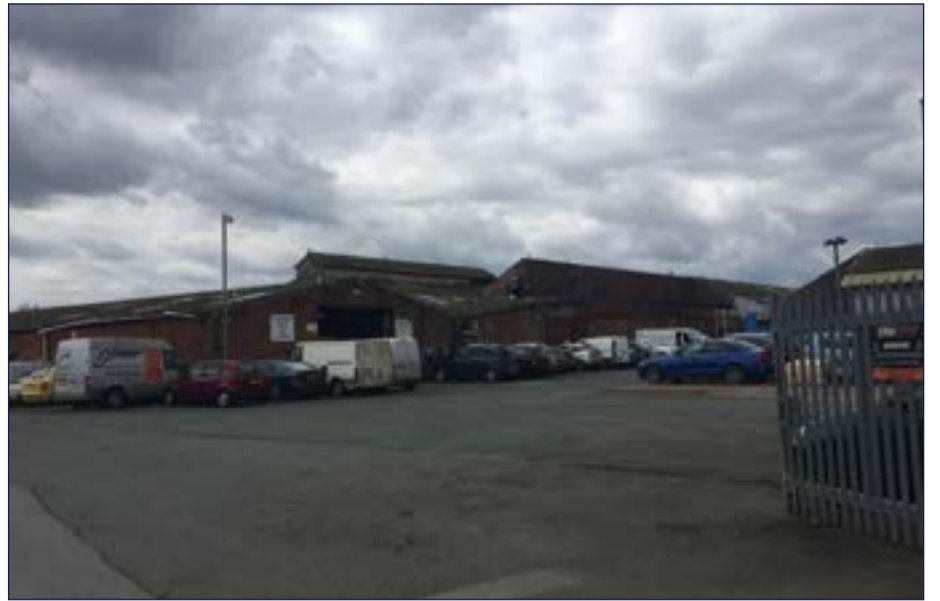
Figure 3.21: Photograph 17 - Water Lane looking towards Vulcan Works buildings
