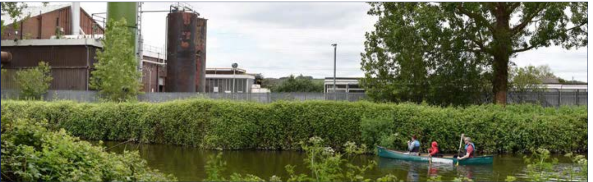
Figure 3.34: Viewpoint from canal looking south towards existing buildings on site [GLA].
