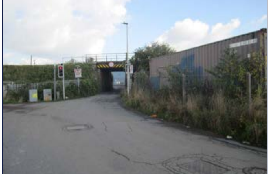
Figure 3.24: Photograph 20 - Tan Lane looking towards railway underpass
