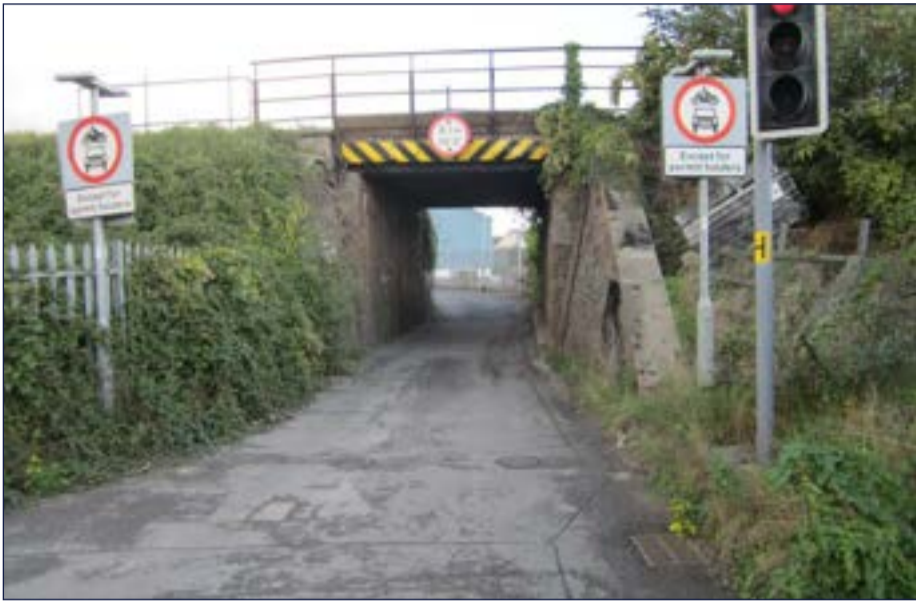
Figure 3.25: Photograph 21 - Tan Lane railway underpass looking south
