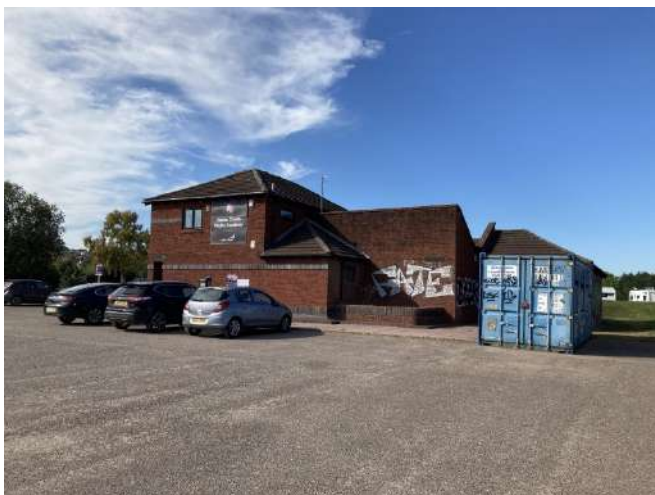
Photo 3: Building B1 (Southern elevation)
