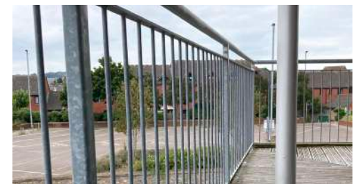
4. Galvanised Balustrade & Steelwork
