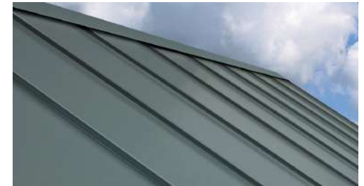
3. Standing Seam Roof
