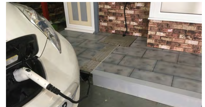
Figure 18 Example of a gully & cable protector
